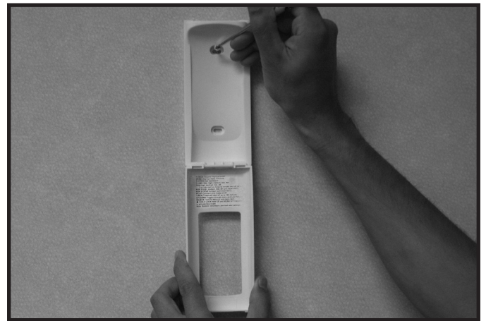
Figure 12.6 Mounting Remote Control Housing
